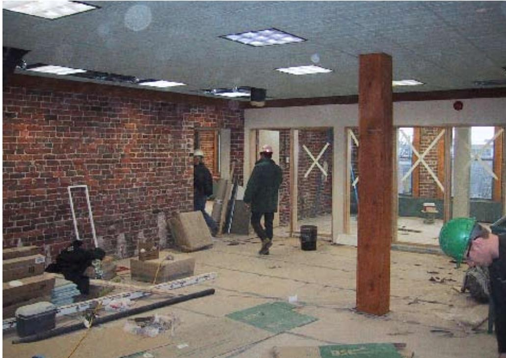
"As well as facilitating the introduction of all new mechanical and electrical systems, we decided to expose the heavy timber and brick bearing wall construction as another way of unifying the project," said Mr. Johnson. "In phase 1 we reinforced everything with great blocks of chunky wood held together with steel straps. We liked the look but, after discussion with Parks Canada, we decided to use more steel in phase two so the original columns can still be seen."
