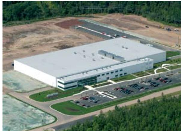
Ocean supplied and installed 710 tons of structural steel, and 230 tons of steel joists in this new state-of-the-art plant. The \$60 million, 150,000 square foot plant produces diapers and training pants and is the first of its kind in Canada.
