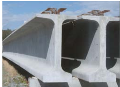
New England Bulb Tee Bridge Girders
