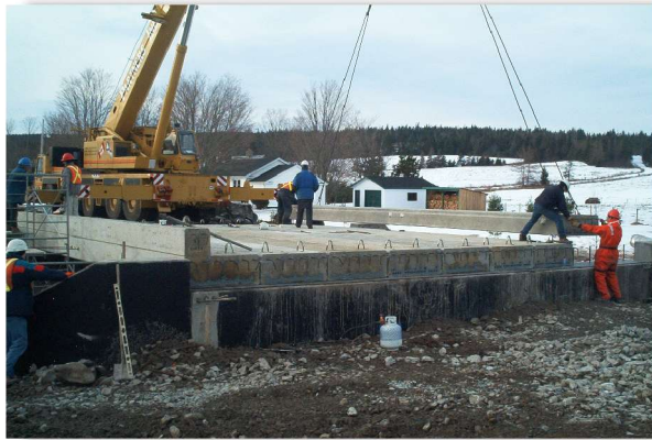
Once all deck slabs are placed the joints will be grouted.
