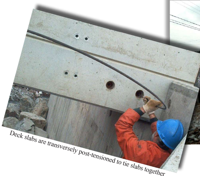
Once all deck slabs are placed the joints will be grouted.
