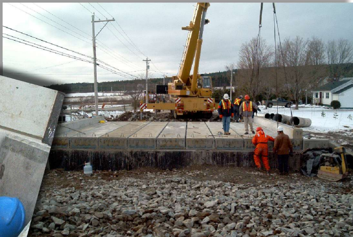
Setting the final Deck slab, with curb, into place.
