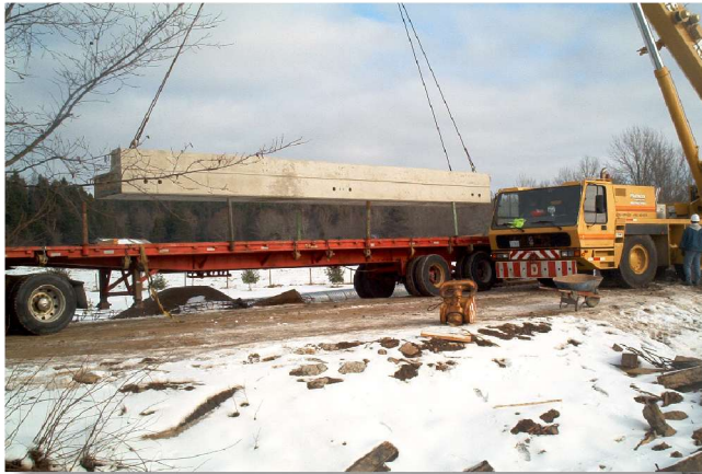
First deck slab arrives on site.
