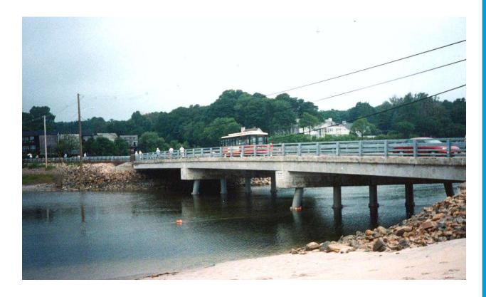
The Department of Transportation used precast prestressed concrete box girders for the bridge at Ogunquit Beach. 33 Box Girders were required that were 31½" (800mm) in depth in 3 - 71 foot spans. Because Ogunquit Beach is a tourist area, the state of Maine wanted a bridge that would not take away from the aesthetics of the beach; therefore a bridge made with precast concrete girders was an appropriate solution.
