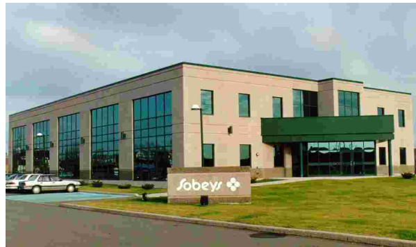
Old Sobeys's Office Building
